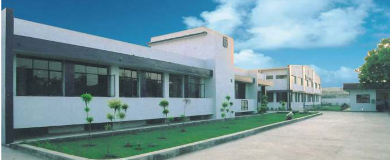
Roto's Manufacturing Plant
